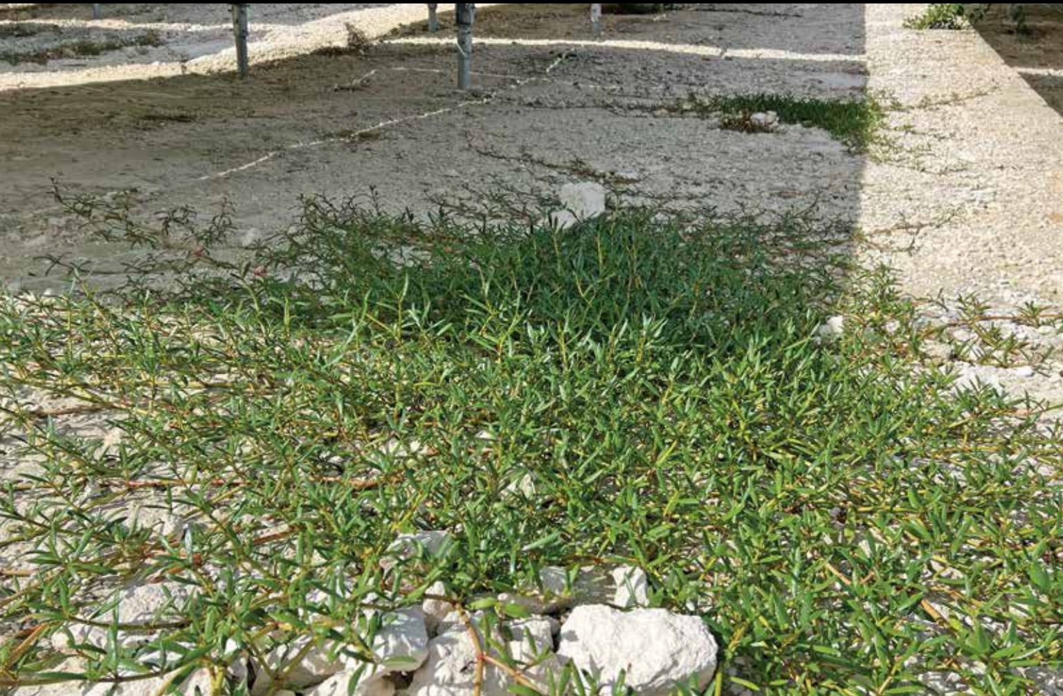
▲ Solar Island Energy plants this sea purslane to help manage the vegetation growth around the PV array and reduce ongoing O&M costs.
